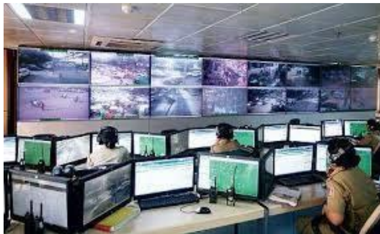
Figure 6. Integrated Command and Control Centre (ICCC)
